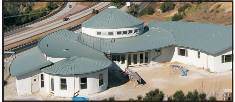
Exterior View of Friends Center November 2008 Photo: Alvin Stern
