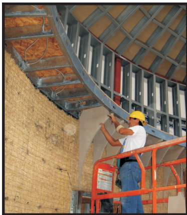
Volunteer Jack Leshefka on the lift setting "ribs" in the Friends Meeting Room. Photo: Wayne Reed
