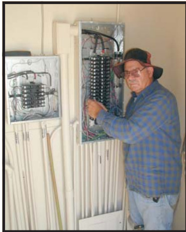
Volunteer Ken Aeschbacher connecting an electrical circuit.
